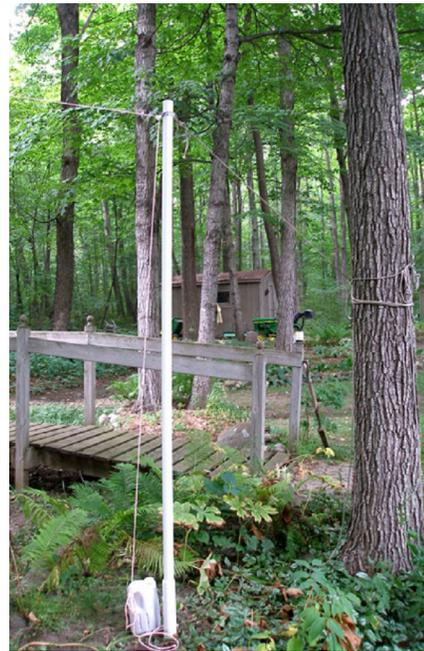
The receiving antenna performance can vary with "ground" conditions so a good ground is required. I used an 8ft. 3/8" copper rod and installed it using a home made driving cap pipe.
