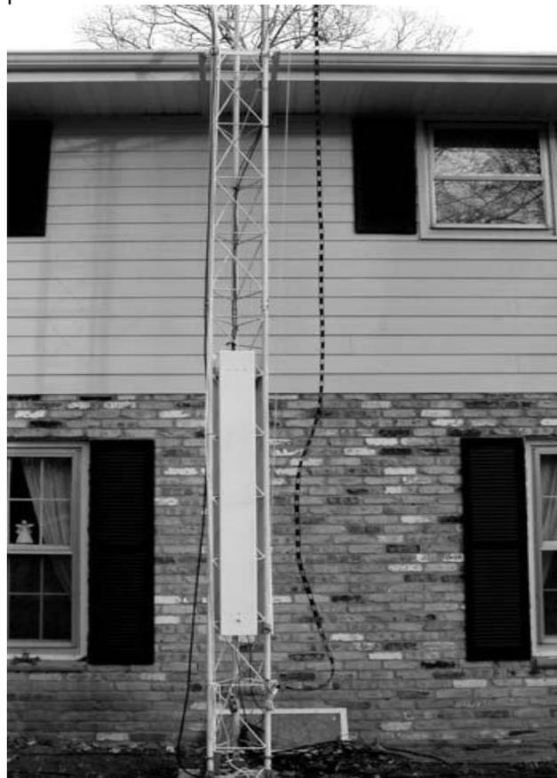
Climbing shields installed on W9IPR's tower. They are recommended if you have a tower and there are curious "kids" in the area.
