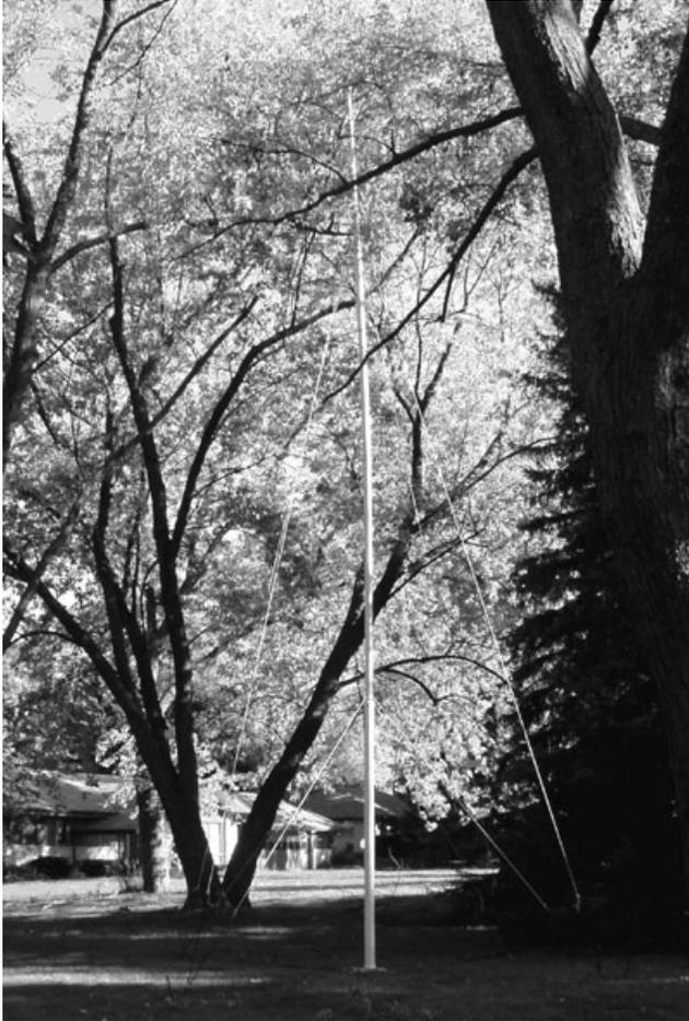
**This is Mark's (KC9GST) newly designed 35 ft. Portable mast made of PVC pipe, a special surface mounting plate, 4 radial support pipes and guy ropes.**
