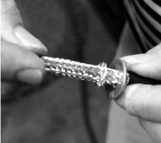
Place the washer at the point on the shield where you intend to make the cut. Then push the shield up against the washer creating a flange.
