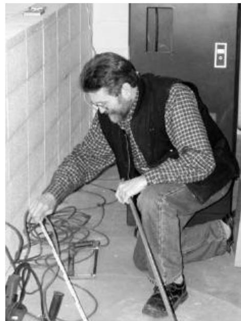
Peter (KB9URH) Schmidt of Schmidt Electric is shown here measuring and cutting conduit in the completion of this repeater site – electrical hook-up.
