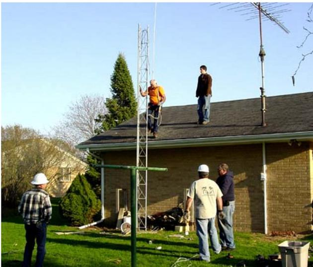
**Almost finished. After the beams, mast and rotor were removed the upper section was jacked apart and again, lowered using the gin pole.**
