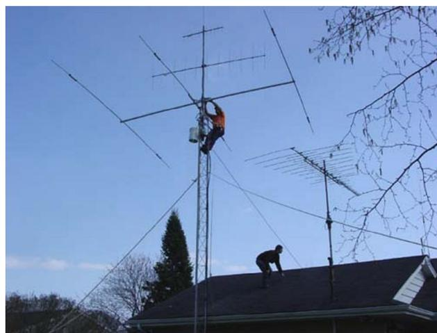
Starting with the TA-33, the beams have to be removed first. Naturally there were a few unique aspects to the installation that slowed
