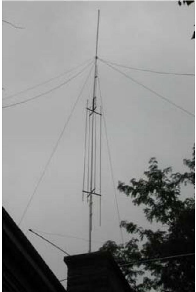
Outside Vic is running a GAP Titan DX with the tuned counterpoise on HF and a Comet dual bander on VHF. He also enjoys going to their cabin near Crivitz where he uses an ICOM 706 to a G5RV on HF and his ICOM W32A HT to work their repeater.
