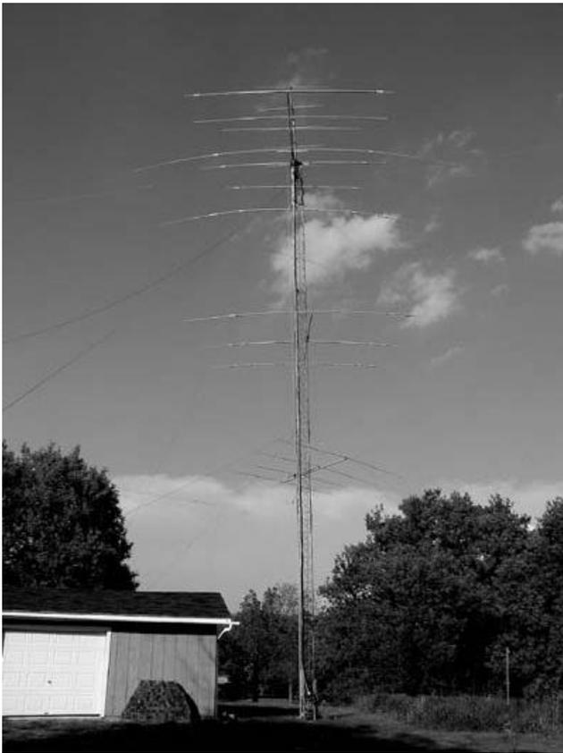
This is one of Fred's two towers used to support the 70cm through 20mtr beams and provide supports for the various slopers, dipoles, long wires and bazookas.
