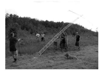
The manual erection of towers was greatly eased due to the use of the hinged base plates as designed and fabricated by Mark Potash (KC9GST)
