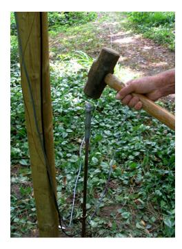
The receiving antenna performance can vary with "ground" conditions so a good ground is required. I used an 8ft. 3/8" copper rod and installed it using a home made driving cap pipe.
