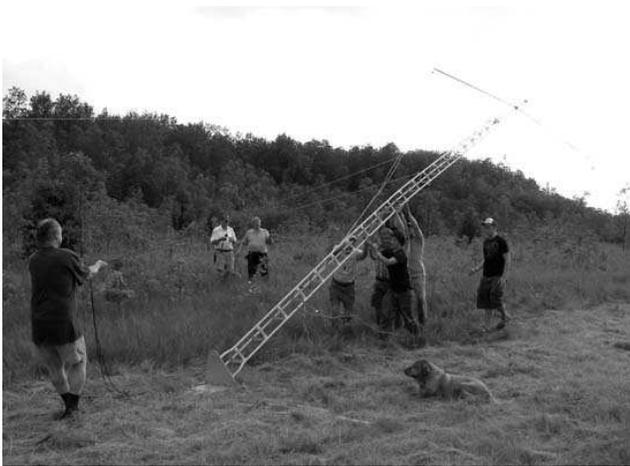
**The manual erection of towers was greatly eased due to the use of the hinged base plates as designed and fabricated by Mark Potash (KC9GST)**
