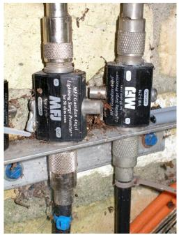
The lightning arresters are fed through a grounded aluminum angle iron for secure protection.
