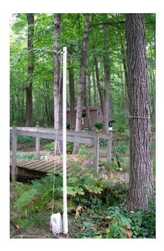
A 2 ft length of PVC pipe was put into the ground to act as a socket for the 8 ft length of PVC pipe used to support the loop corners. This allows the antenna to be easly disassembled if desired. There is a pully at the top of the pipe and the loop corner is supported by a rope through the pully and weighted by a milk jug filled with sand. This allows the supporting tree to move and sway without stressing the antenna loops.
