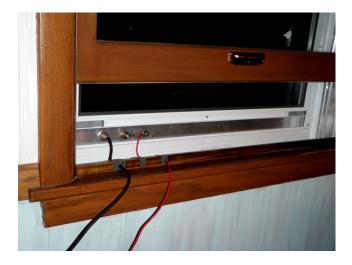
Then a wood spacer was cut to install in the lower portion of the inside window frame. Three ¾' wide slots were cut in the wood spacer and then ½' adhesive backed weather strip was inserted into the slots to form a slit and seal the area through which the antenna coax and ground wire would pass.
