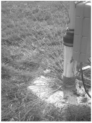
PVC Pipe Mount for Flag Pole Vertical Showing Termination of 120 radials at common ground rod
