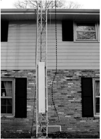
Climbing shields installed on W9IPR's tower. They are recommended if you have a tower and there are curious "kids" in the area.
