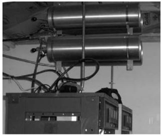
The duplexer (4 pipes in upper part of picture) allows one antenna to receive on one frequency while it transmits simultaneously on a different frequency
