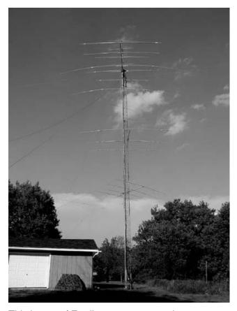
This is one of Fred's two towers used to support the 70cm through 20mtr beams and provide supports for the various slopers, dipoles, long wires and bazookas.
