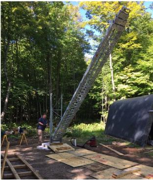
the tower sideways into alignment with the base. A bit of re-rigging with some fulcrum and lever work and we had the tower bolted to the base. We carefully raised it to full extension and back again. A major milestone achieved.
