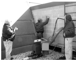
Here Mark Potash (KC9GST) attaches one of the antennas mounting brackets he fabricated to the firehouse wall while Gabe Chido (WI9GC) and Tom Oehler (W9LNL) supervise.
