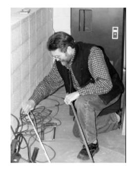
Peter (KB9URH) Schmidt of Schmidt Electric is shown here measuring and cutting conduit in the completion of this repeater site – electrical hook-up.
