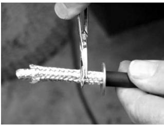
Use manicure scissors to trim around the shield at the base of the flange and then slide off the excess shield.
